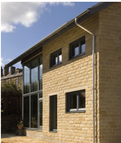
© Green Building Store
